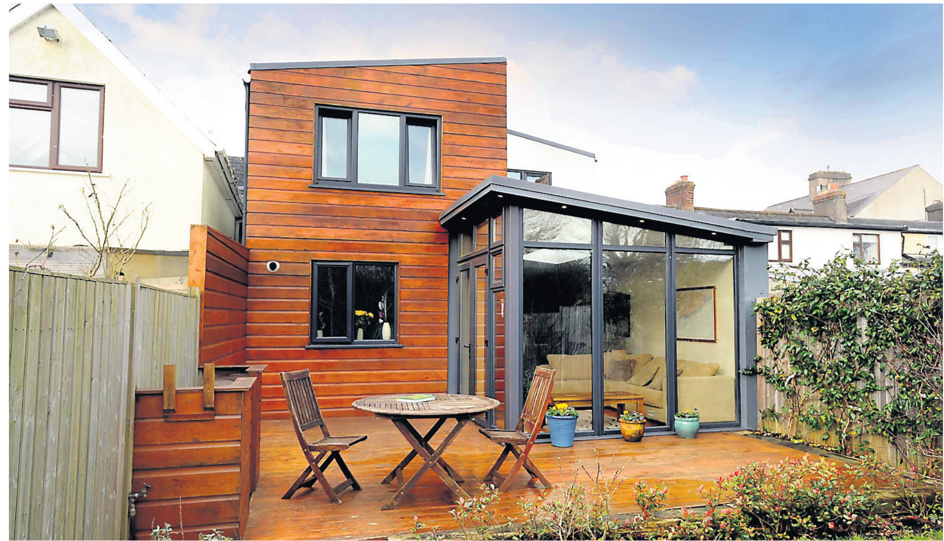
The rear elevation of extension showing integration with deck and garden.
