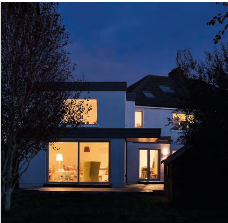
BELOW: An evening view of the house; the complex and stacked extension is easily read from the rear. Pic: Jan O'Connell
